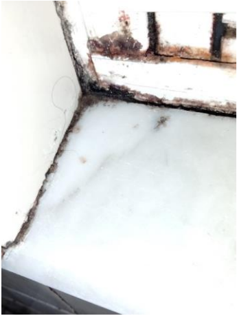
Mold on walls after they were washed with bleach
