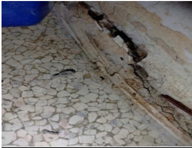
Crack in foundation
